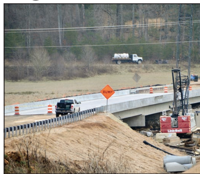
The new SR 66 bridge over Brasstown Creek is now in service. Just watch out for that bump. Photo by Jarrett Whitener
